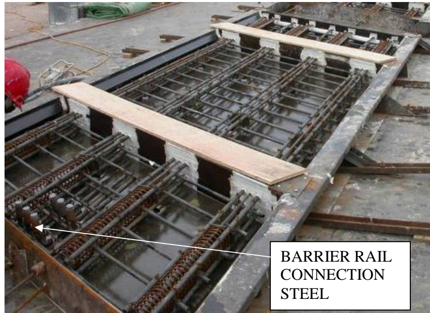
a) deck panel reinforcing steel
