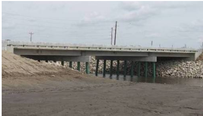
b) completed replacement bridge
