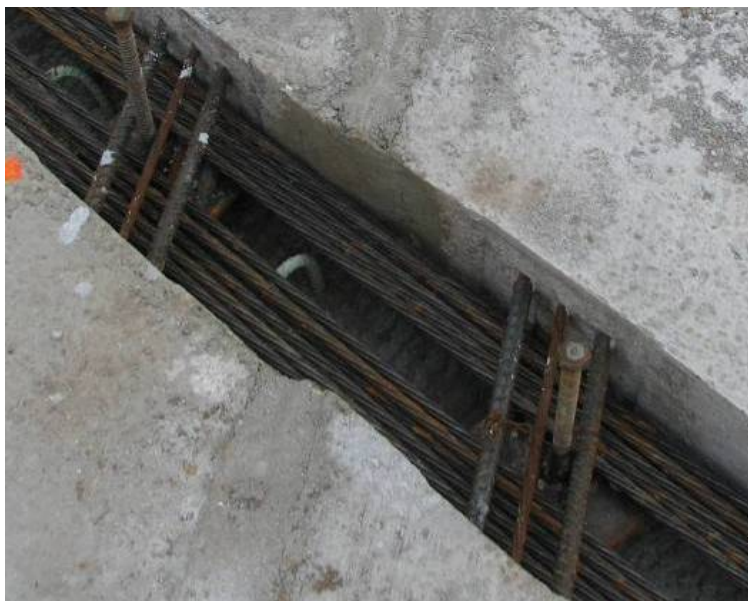
Figure 2.17. Photograph of longitudinal post-tensioning channel prior to casting concrete in the field.
