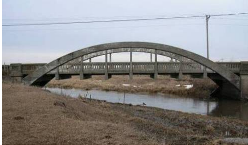
a) replaced Marsh Arch bridge
