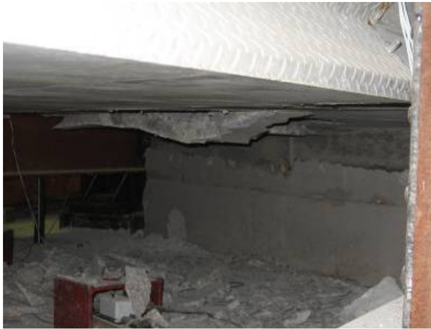
c) underside of the deck panel
