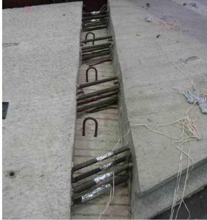
Figure 2.10. Reinforcing bars instrumented with steel strain gages.
