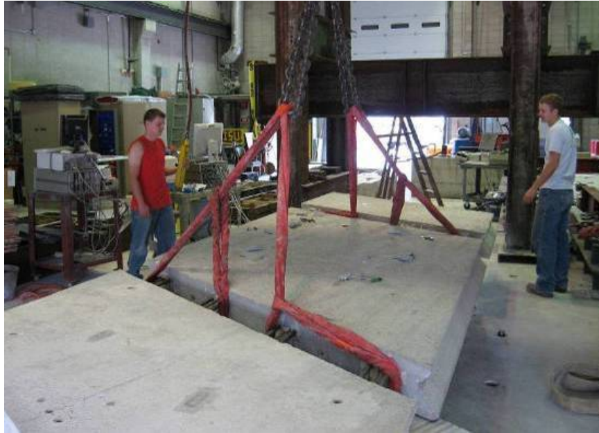
a) photograph of lifting the deck panel with four straps
