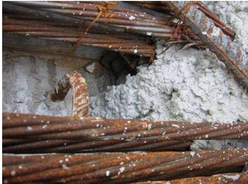
b) concrete flowing between post-tensioning strands
