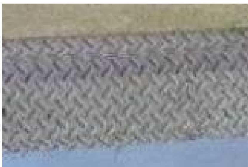
Figure 2.3. Textured surface of transverse joint.
