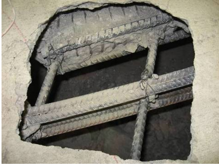
b) top view after concrete removal
