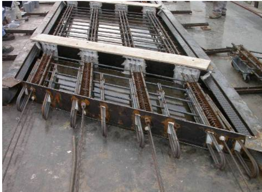
b) double hooks and prestressing strands
